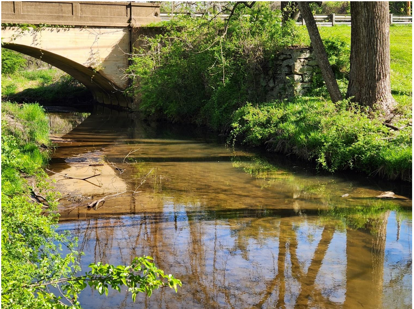
Figure 1 – Brice Run at Old Court Rd and the original Bridge Abutment
