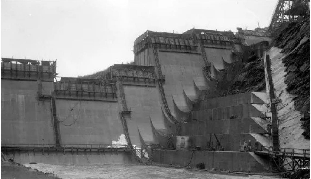
The Dam Under Construction
