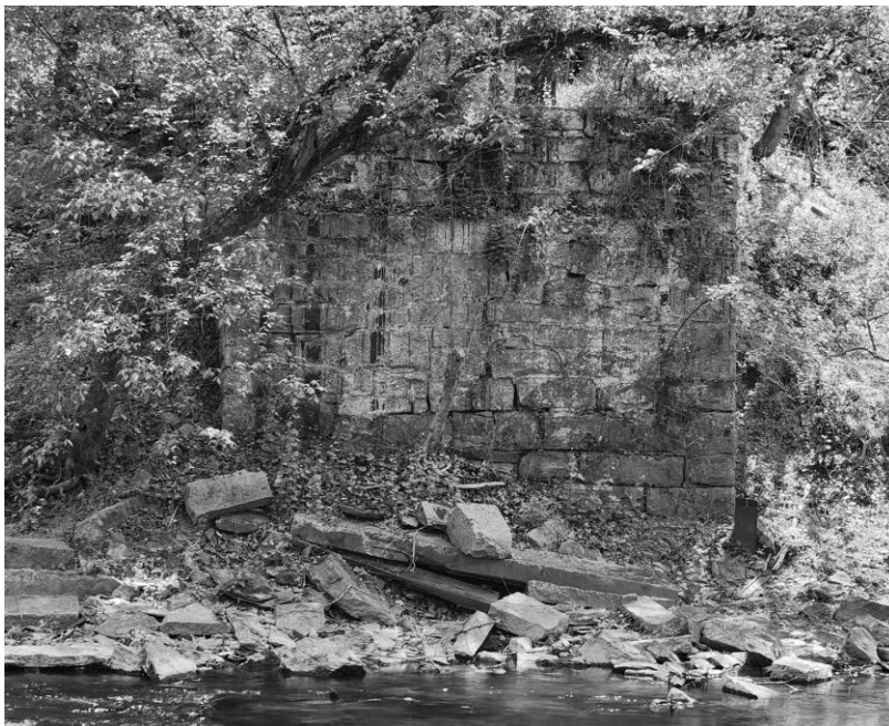
Remains of the abutment on Howard County side of the river, 2023
